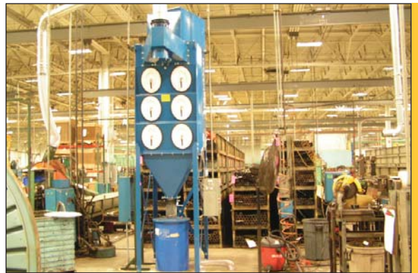
DFO 3-6 on sawing of high pressure hydraulic hose
