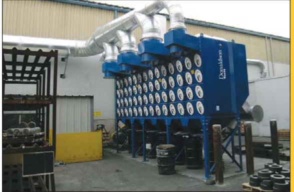
DFO 4-112 on titanium grinding
