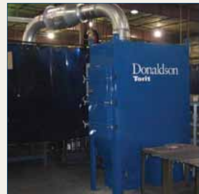
TG4 on welding
