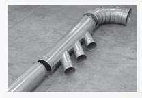
**STEP FOUR:** Laying out the duct. Begin by laying the system out on the floor below where it will hang. Remember that two parts that connect will often not be in the same box, so this step dramatically reduces the time it takes to complete the job once the installation begins.
