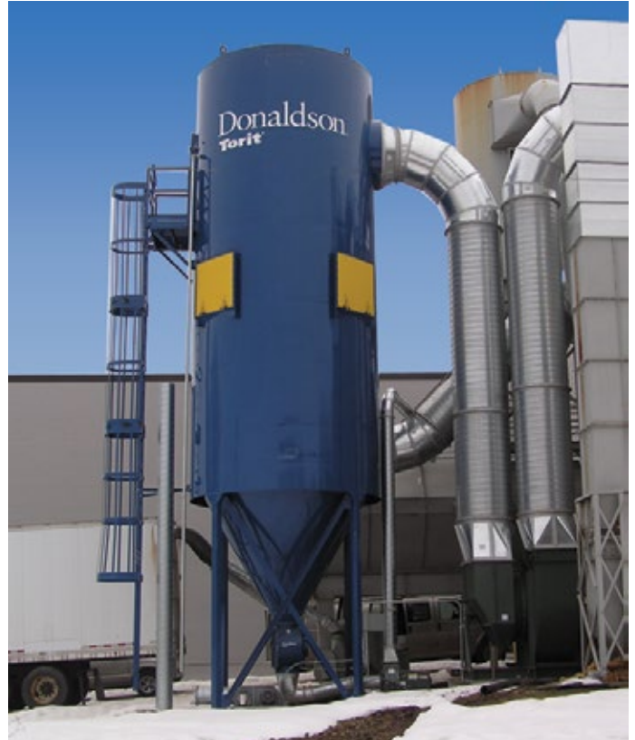
376RF at Cabinet Shop
