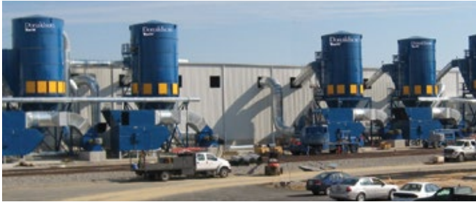
776RF at Wood Furniture Plant
